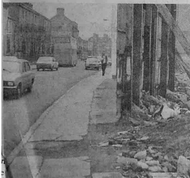
GONE . . . a derelict site cleared for the roadway project.
